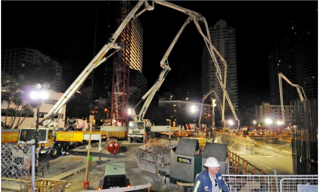
Construction of Panorama Tower, 1101 Brickell Ave.
