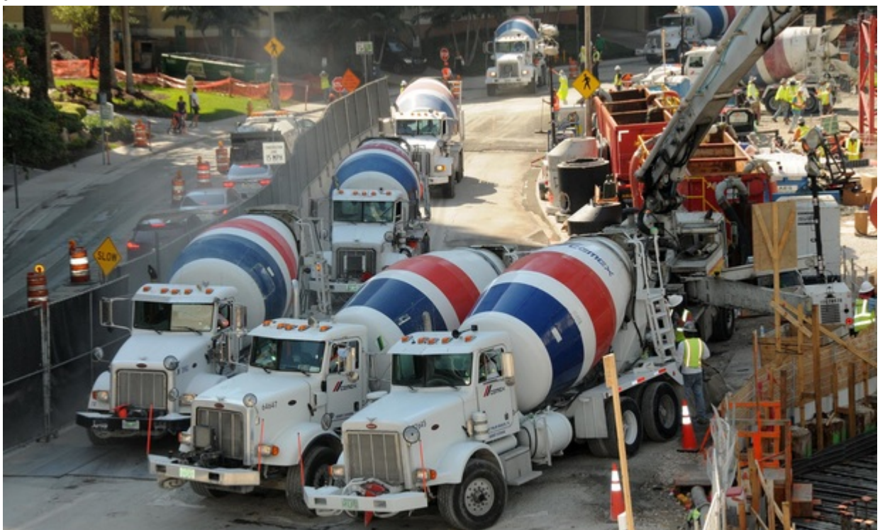
Construction of Panorama Tower, 1101 Brickell Ave.
