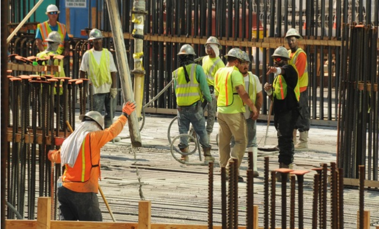
Construction of Panorama Tower, 1101 Brickell Ave.
