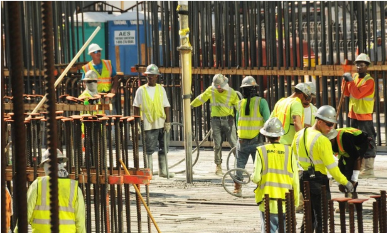
Construction of Panorama Tower, 1101 Brickell Ave.
