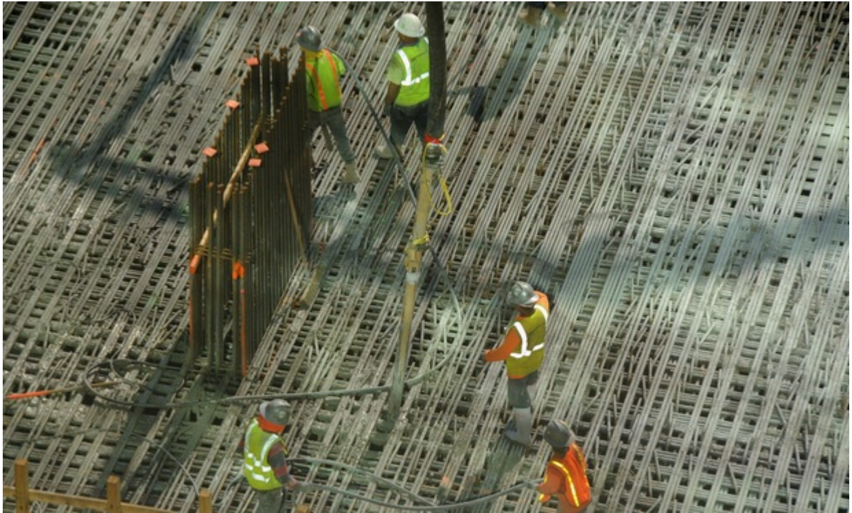
Construction of Panorama Tower, 1101 Brickell Ave.
