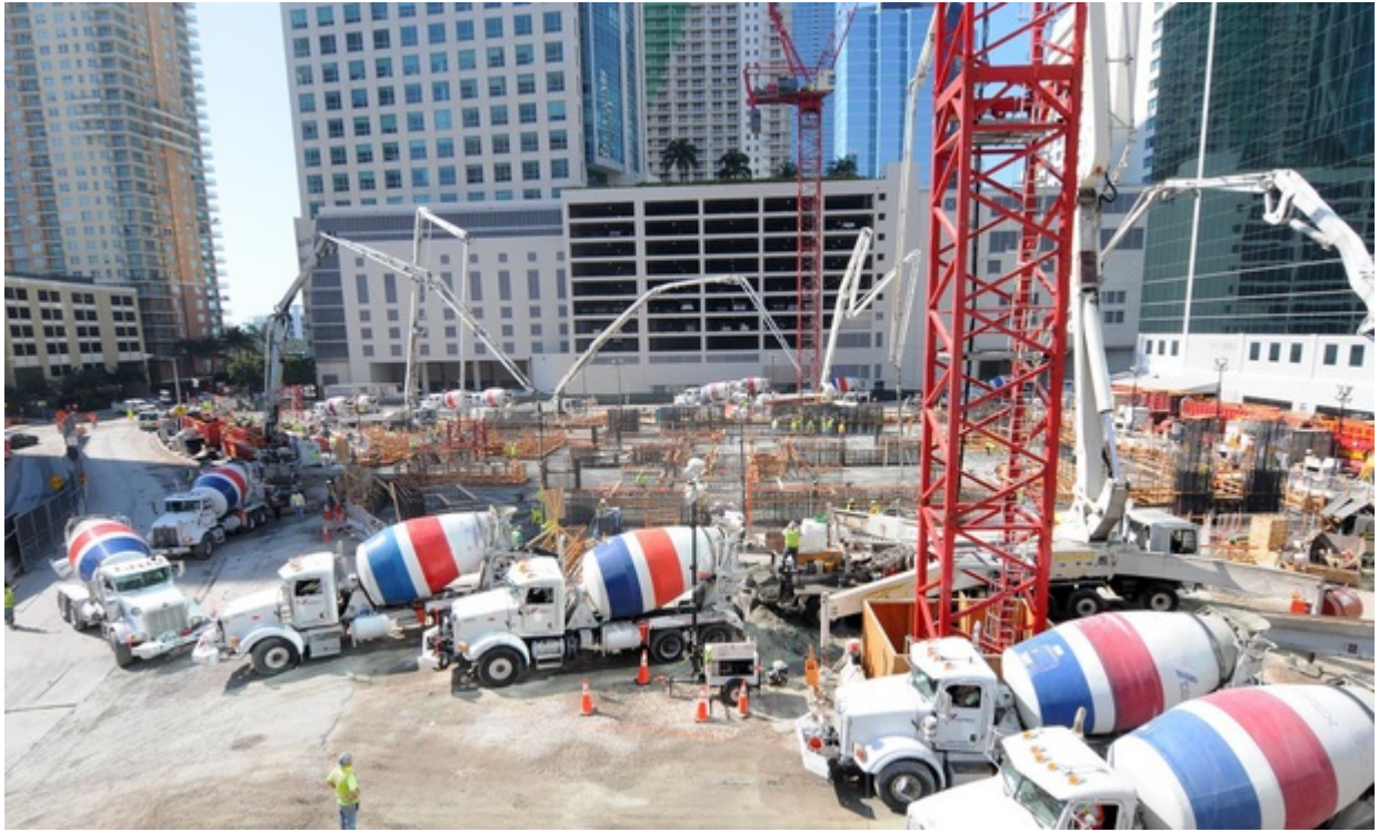
Construction of Panorama Tower, 1101 Brickell Ave.
