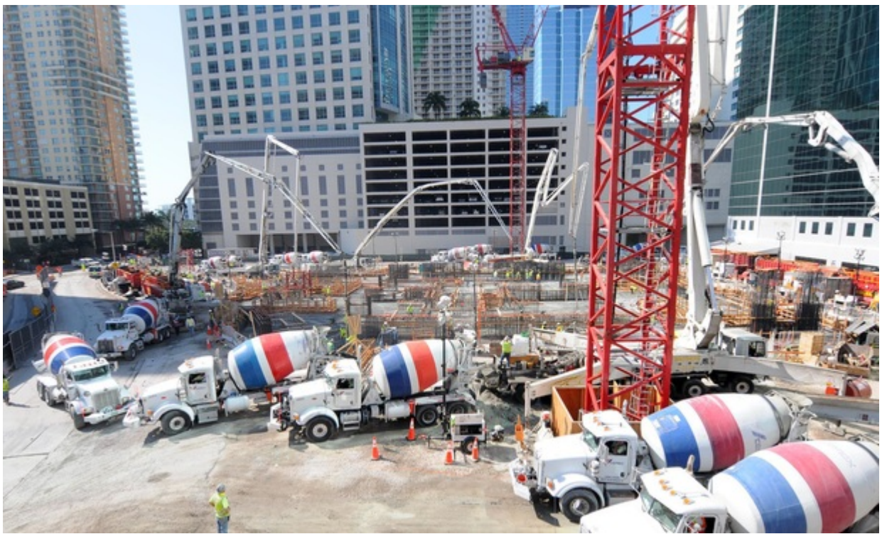
Construction of Panorama Tower, 1101 Brickell Ave.
