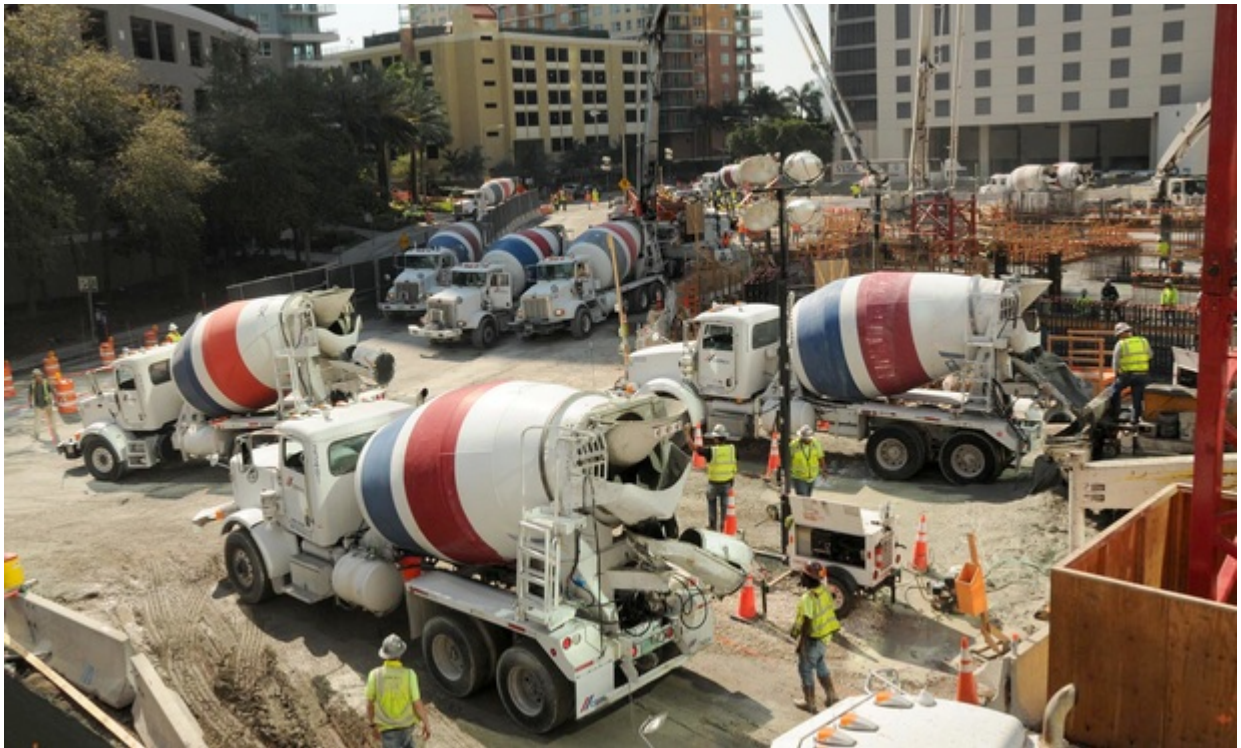
Construction of Panorama Tower, 1101 Brickell Ave.
