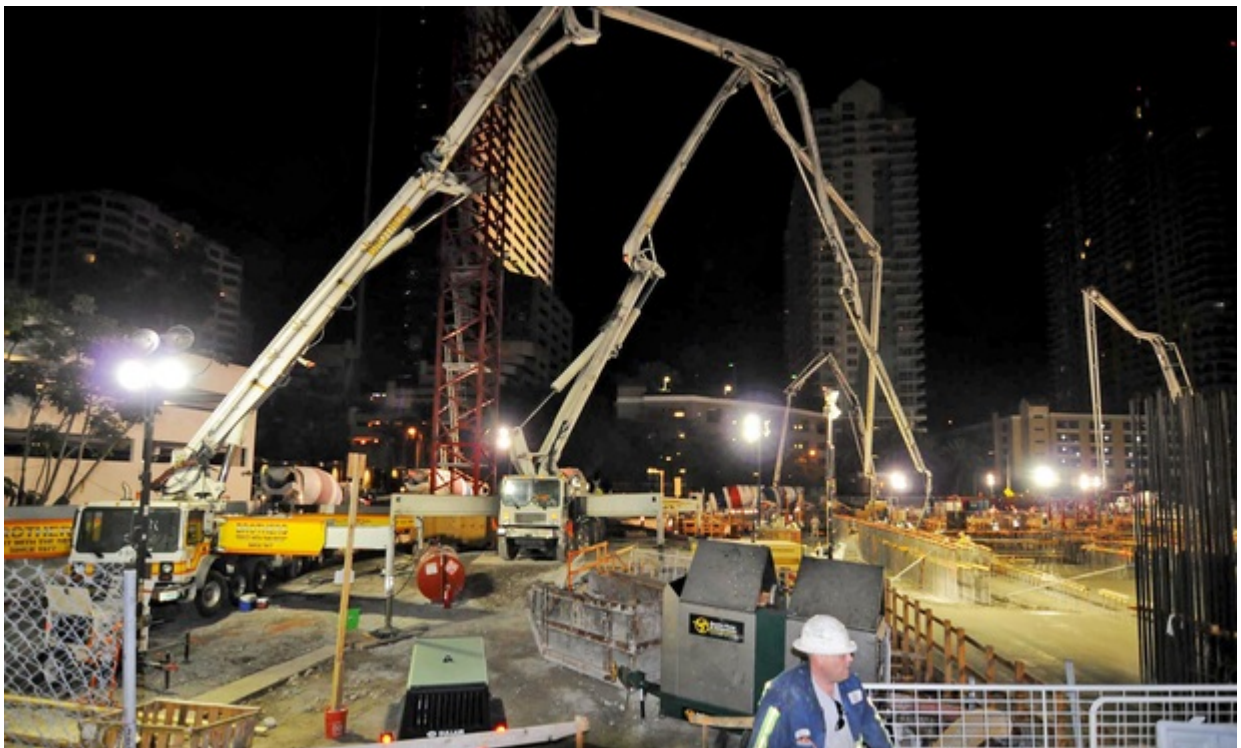
Construction of Panorama Tower, 1101 Brickell Ave.
